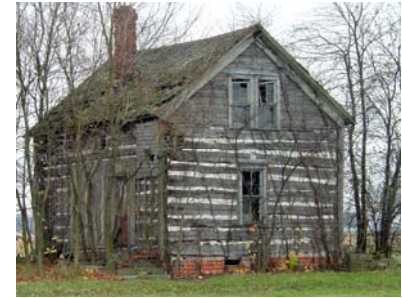
A neglected log house located on US 24 east of New Haven; it is adjacent to the former Wabash & Erie Canal, and within the potential Maumee River Heritage Corridor.
